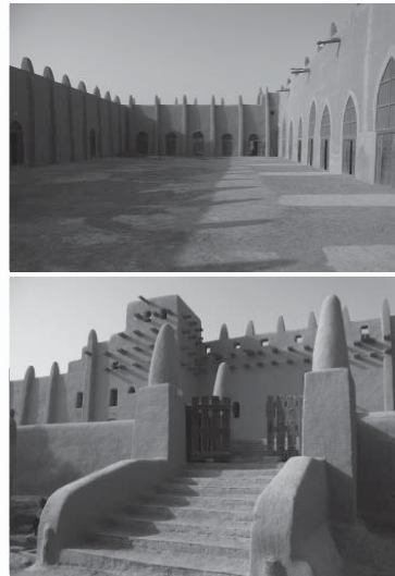
Pict. 7, 8 Mosque Restoration (Roof) Source: Oussouby SACKO (2010.2)
