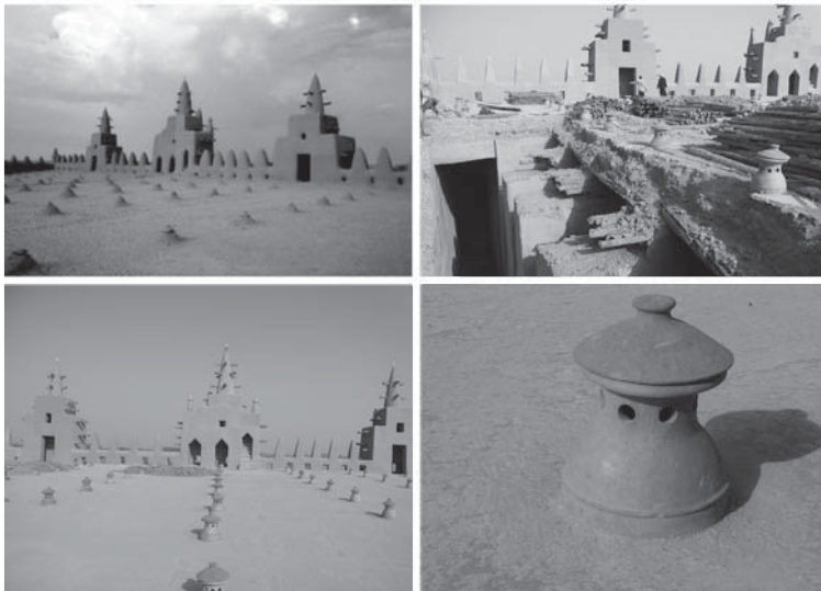
Pict. 9, 10, 11, 12 Roof top light renovation Source: Oussouby SACKO (2004.5, 2010.2)
