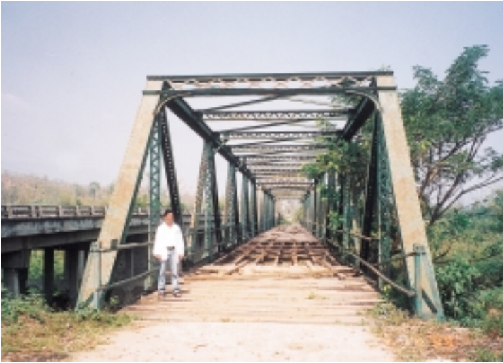
(7) Bridge over the River Pai.
